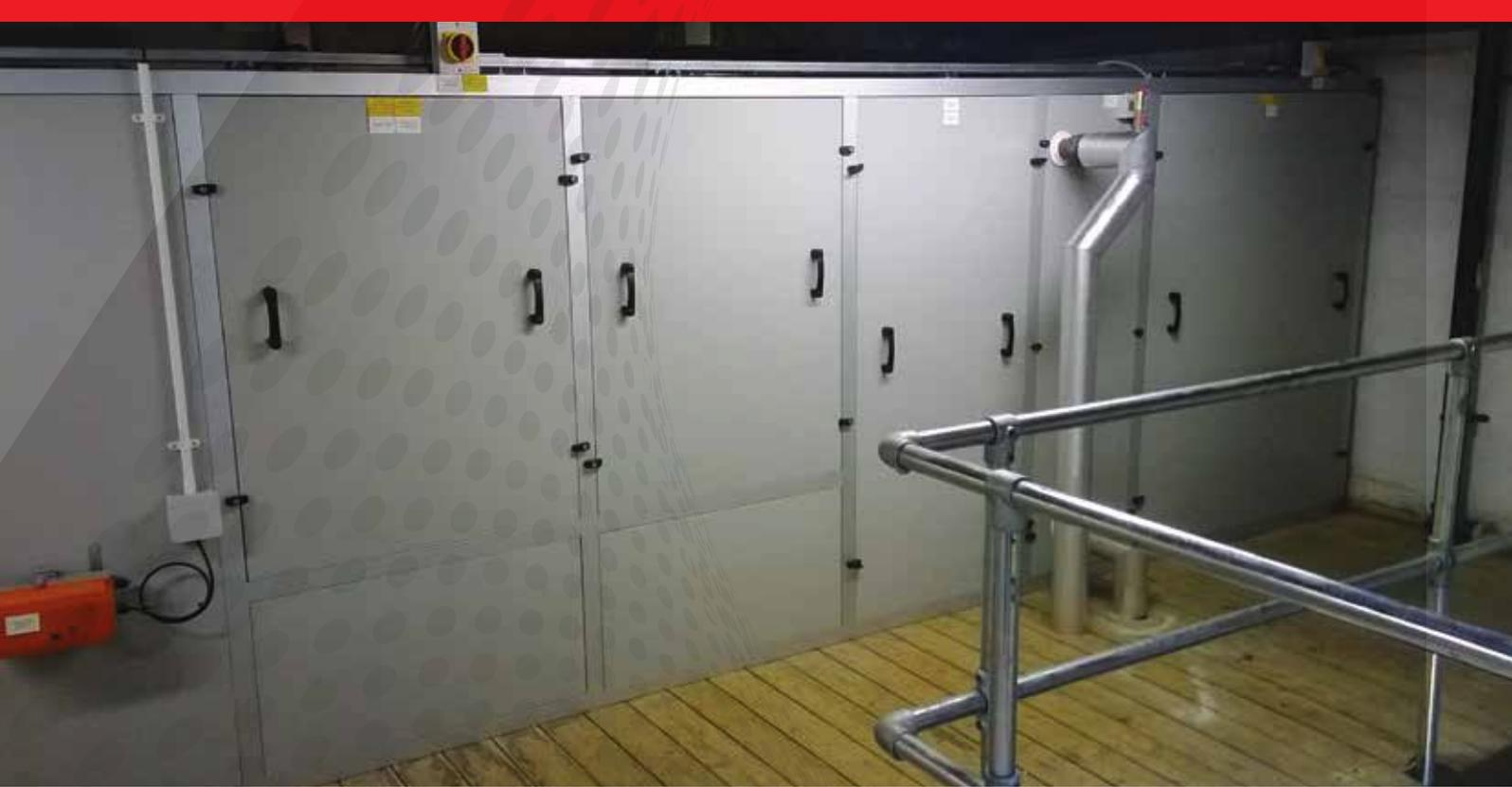
The air handling unit (AHU) was shipped to site in component form and assembled in position on a mezzanine floor in the existing pool plant room. The AHU includes three energy conservation systems, variable fresh air ventilation, plate heat exchanger heat recovery and variable rate ventilation control. This provided an energy savings of approximately 75% and a carbon reduction of approximately 230 tonnes a year compared to the original full fresh air system it replaced.
